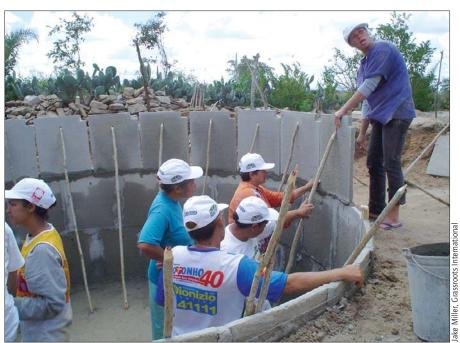
Installing a cistern to capture rain for irrigation and drinking water in Brazil's arid Northeast
