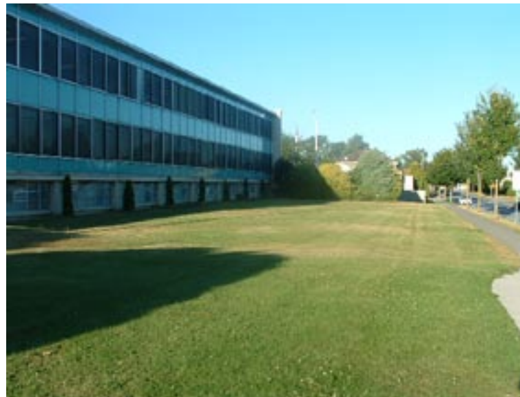
Pilot Site #3: View Facing East
